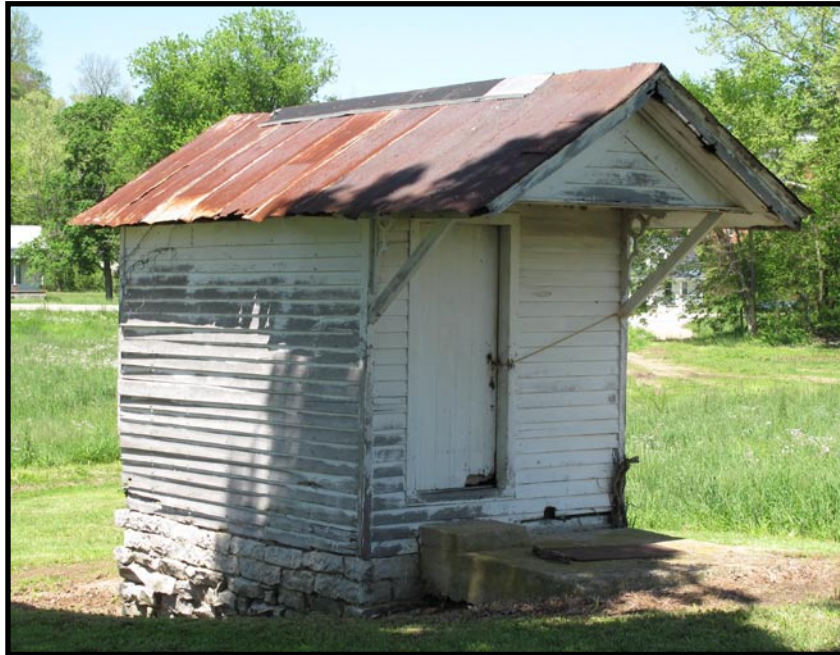
Figure 143 Springhouse and dry storage at the Pryor Prewitt House, CS-10, Ellisburg quad. Cistern access is in front, to right of door.
