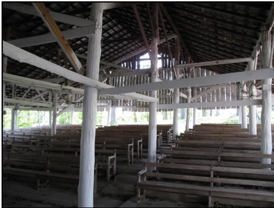
Figure 5. 40 Interior of the Hurricane Shed (CN-25).
