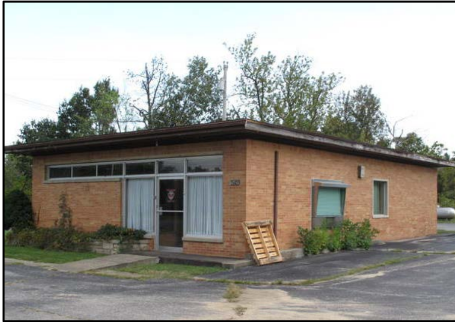
Figure 5. 19 Former bank building (LV-93) in Tiline.
