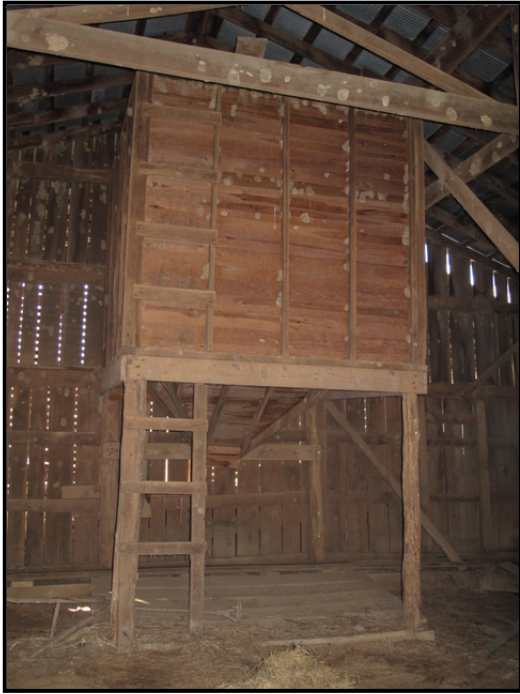
Figure 3. 38 Interior silo, CN-31.
