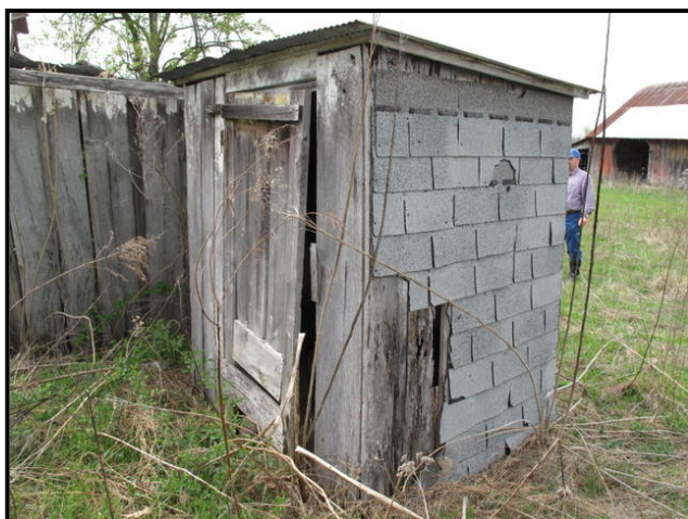
Figure 4. 38 Privy at LV-68.
