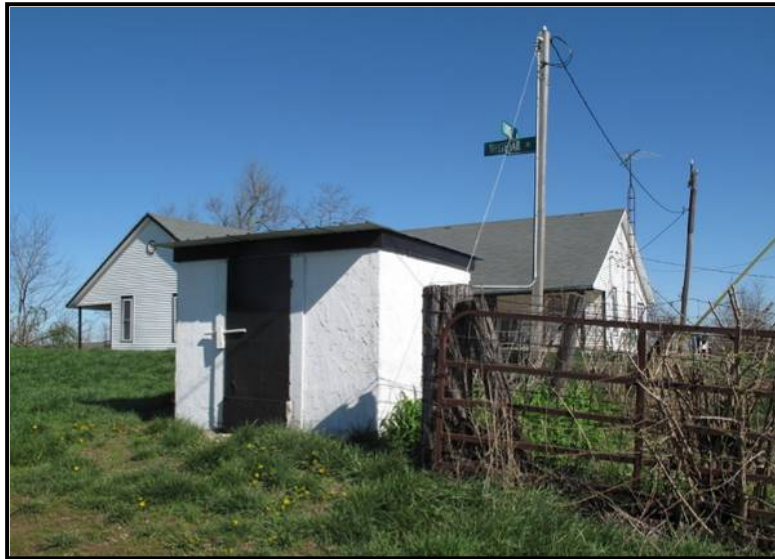
Figure 4. 35 Concrete pump house at CN-31.
