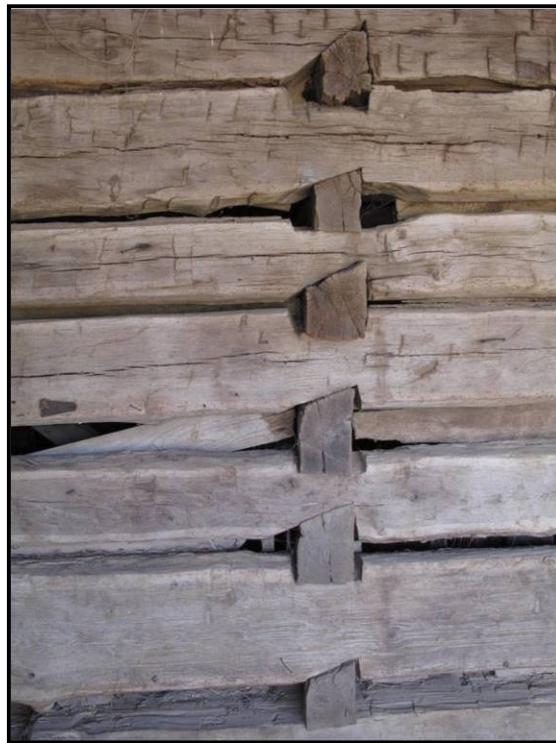
Figure 3. 13 Detail of notching on log crib, CN-63.
