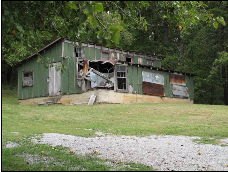
Figure 4. 19 Half-monitor chicken house at LV-87. This type of house was more expensive to construct than a simple shed roof version. Widely touted by agricultural colleges in the 1920s and 1930s, the plan typically ranged from 20 feet wide to 18 feet long.
