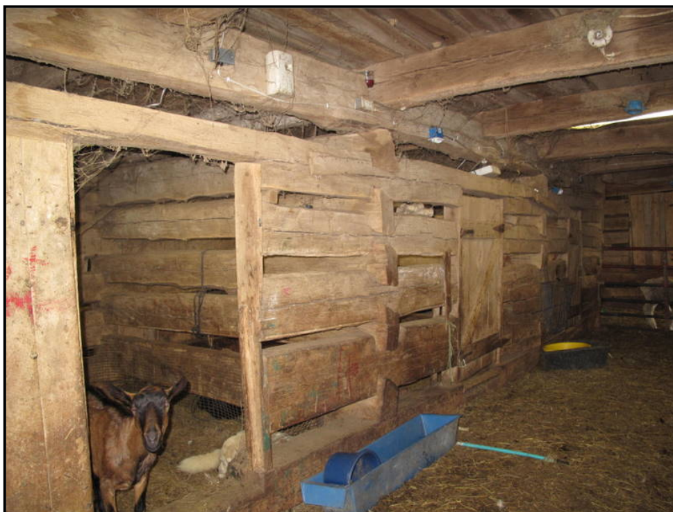
Figure 3. 14 Log stalls on the west side of the barn, CN-63.
