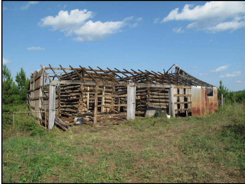
Figure 3. 15 Log barn (CN-70), now demolished, on Route 91 in Crittenden County.
