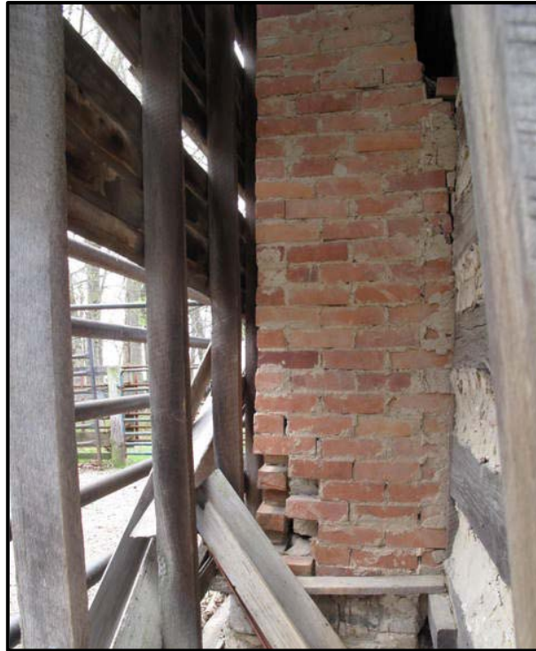
Figure 6. 8 Stack behind framed wall.
