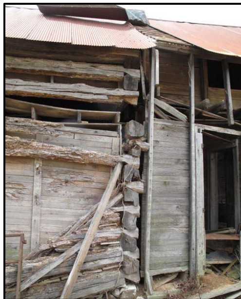
Figure 6. 5 Intersection between the log and frame pens, LV-65.
