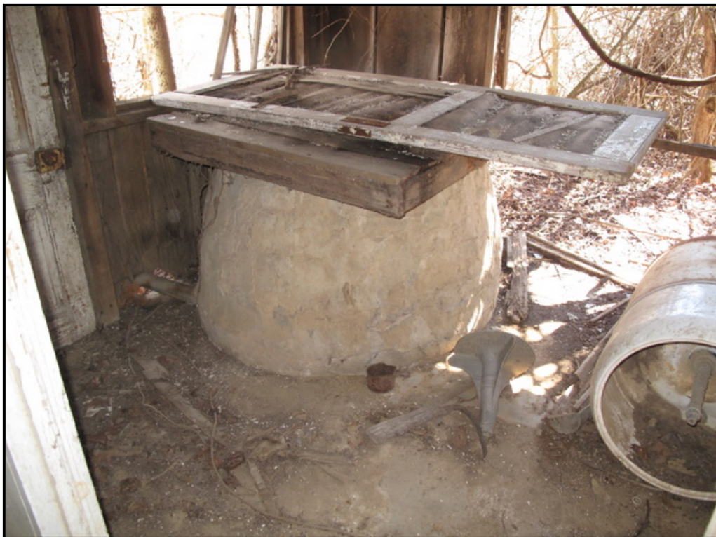
Figure 4. 31 Cistern on enclosed porch at CN-31.
