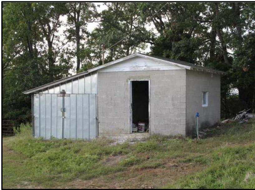
Figure 5. 15 Former polling station in Crittenden County, CN-26.
