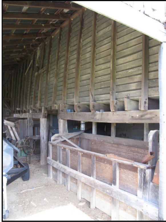
Figure 3. 80 Lower level of LV-54 corncrib.
