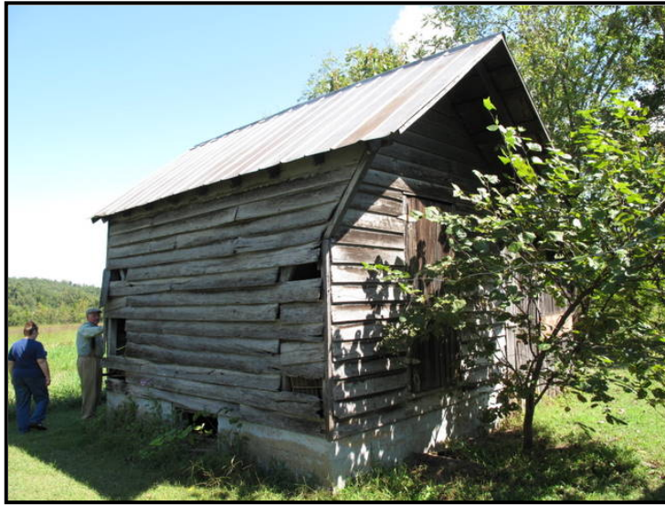
Figure 4. 8 Meathouse/cellar/wash house combination at CN-77.
