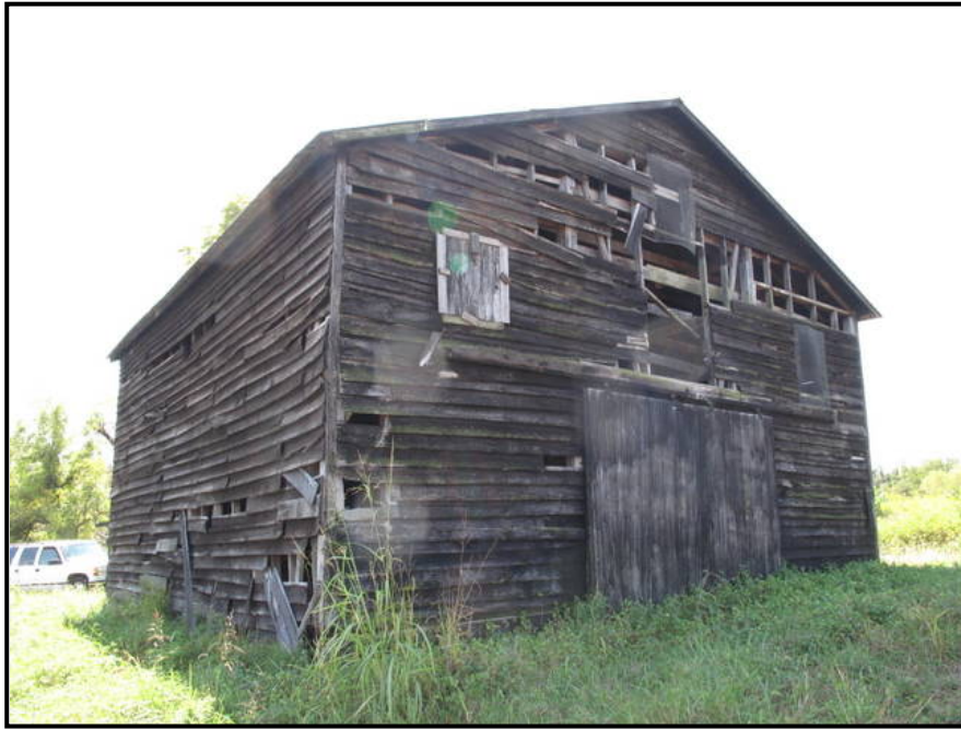
Figure 3. 55 East and north elevations of CN-45.
