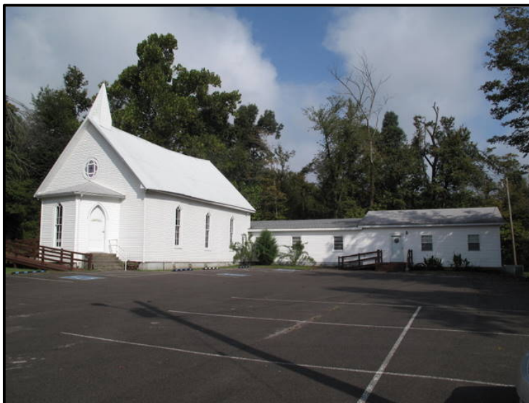
Figure 5. 33 Sulphur Springs Baptist Church (CN-60). Sunday School rooms extend laterally at the rear.
