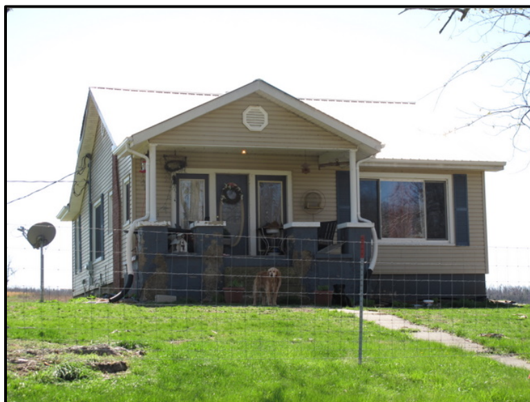
Figure 6. 48 CN-35, a possible Wigginton-built bungalow in Crittenden County.
