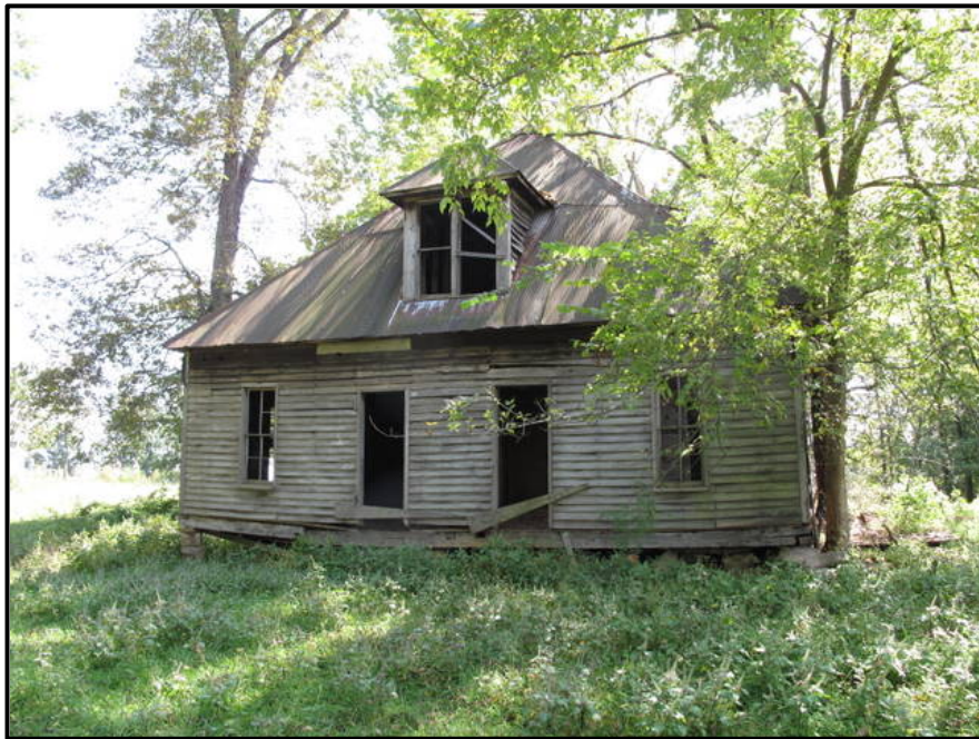
Figure 6. 45 CN-66, a two-front-door house in Crittenden County.
