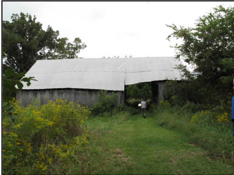
Figure 3. 42 LV-82.3, the second Appalachian Barn at this site.
