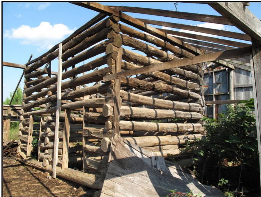
Figure 3. 16 Detail of one of the cribs at CN-70.
