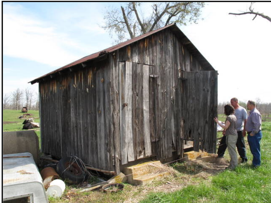
Figure 4. 26 Combination root cellar and storage building, LV-64.
