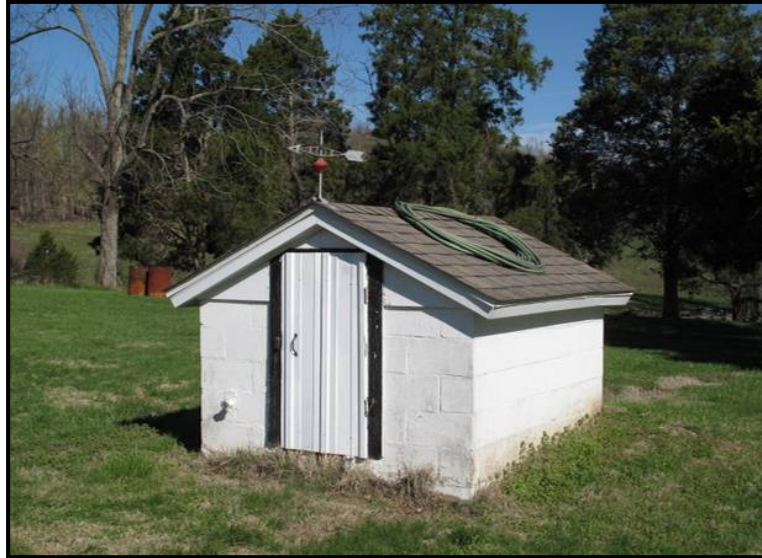
Figure 4. 34 Concrete block pump house at LV-51.
