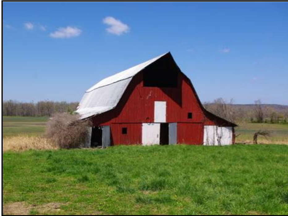
Figure 3. 25 LV-26, a multi-purpose barn on River Road in Livingston County.
