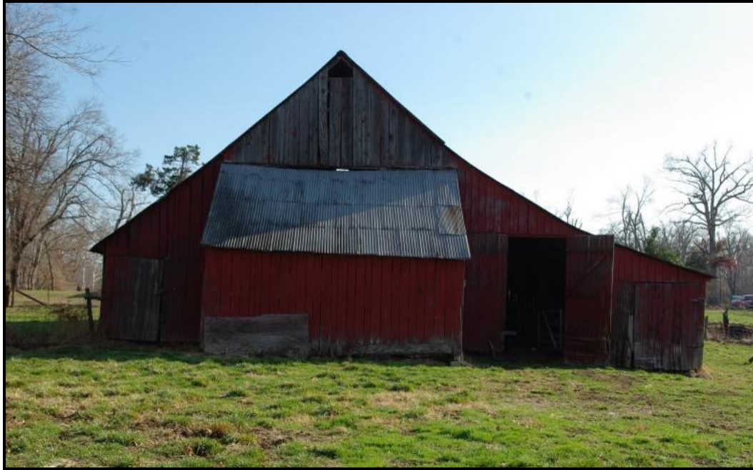
Figure 3. 5 East gable end of barn at LV-42.
