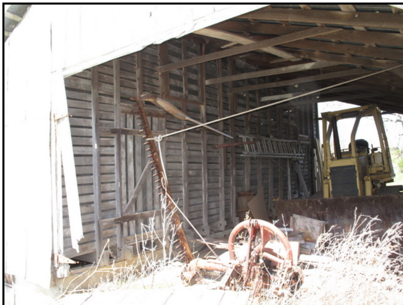
Figure 3. 79 Corncrib at LV-54, upper level.
