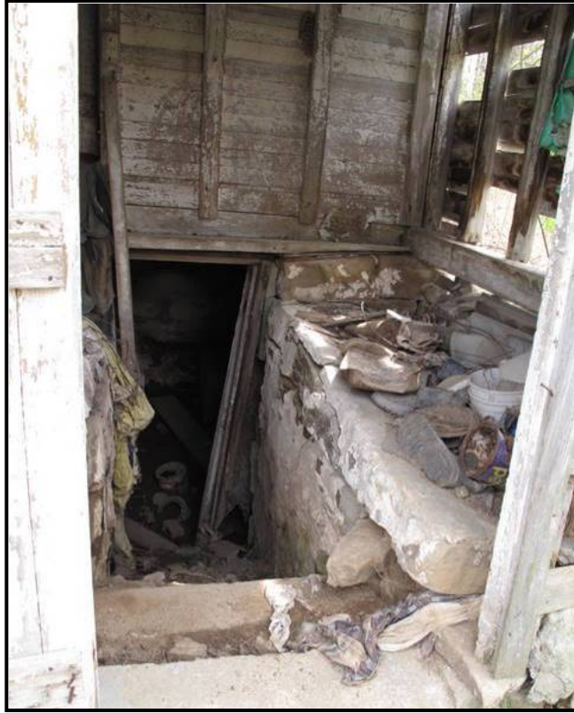
Figure 4. 23 Steps leading down to cellar at LV-68.
