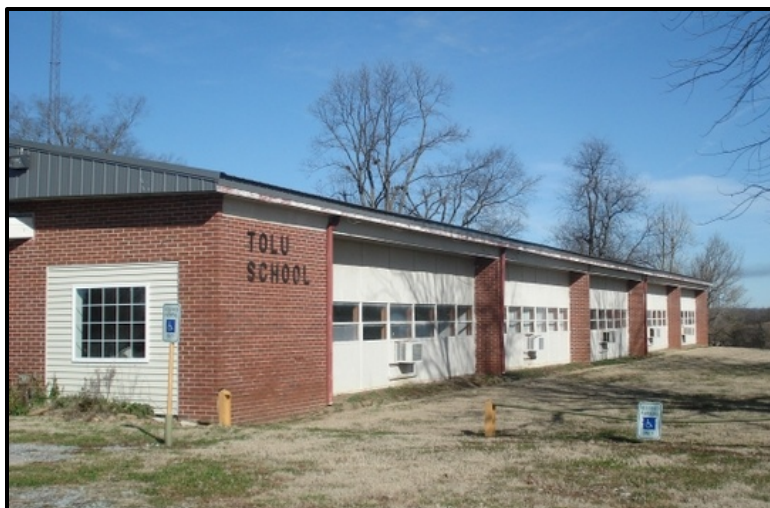
Figure 5. 29 Part of the façade and south elevation of Tolu School (CN-88). Photo by Kathleen Guess.
