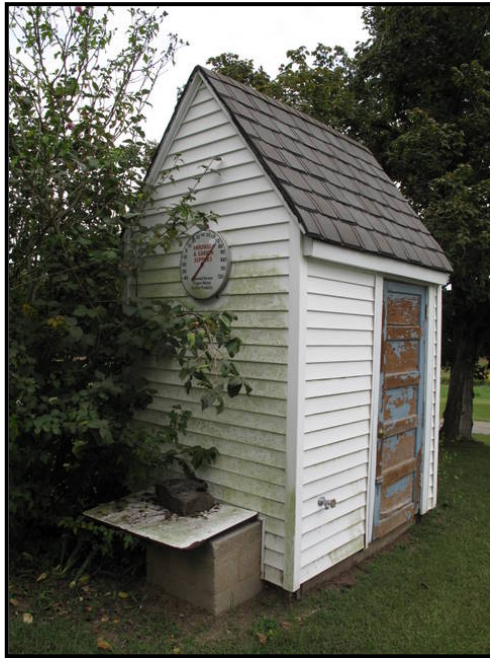
Figure 4. 36 Frame pump house at LV-87.
