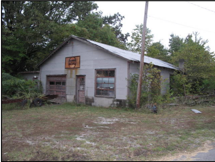
Figure 5. 16 Garage in Frances (CN-56).
