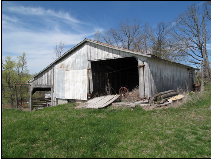
Figure 3. 78 Corncrib at the Old Smith Farm, LV-54.
