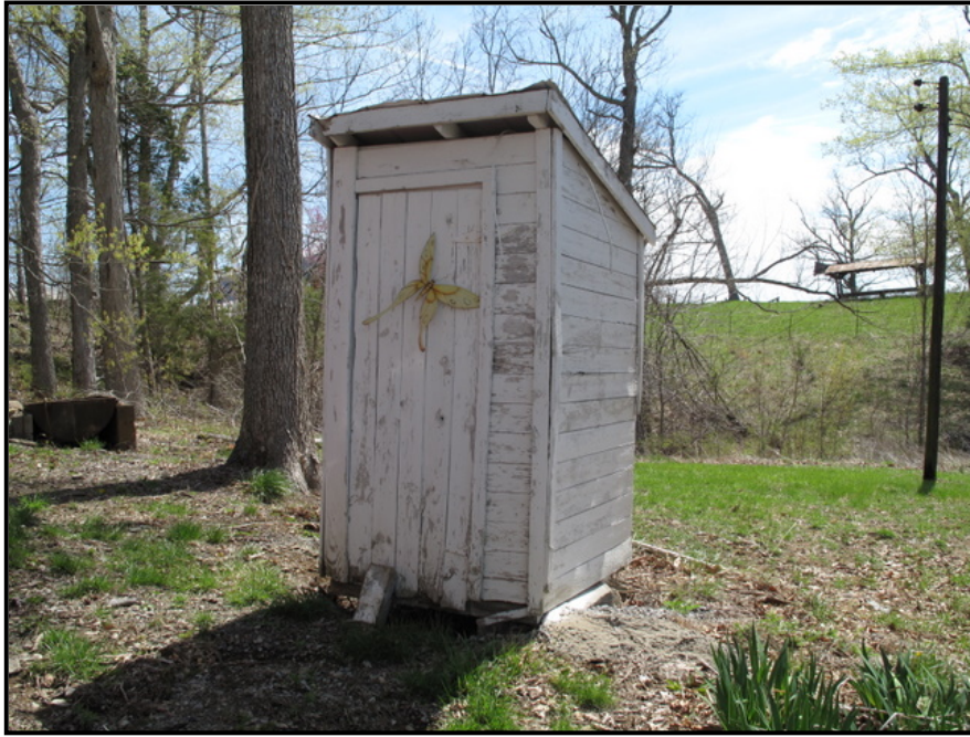
Figure 4. 40 Weatherboarded privy at LV-54.
