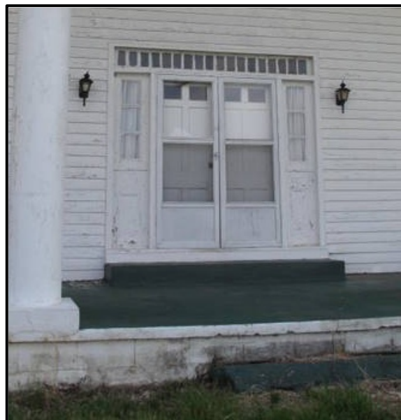
Figure 6. 10 Detail of the doorway at the W.E. Chipps House (LV-73).
