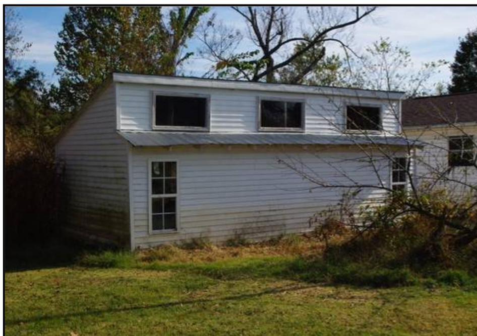
Figure 4. 18 Remodeled chicken house at LV-97 on River Road
