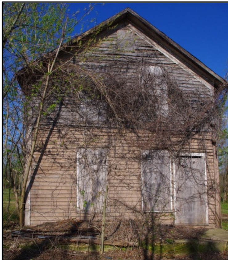
Figure 5. 9 LV-33, an abandoned store in Iuka on the Cumberland River.
