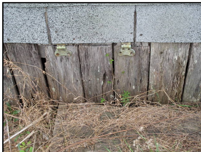
Figure 4. 39 Hinged opening on LV-68 privy.
