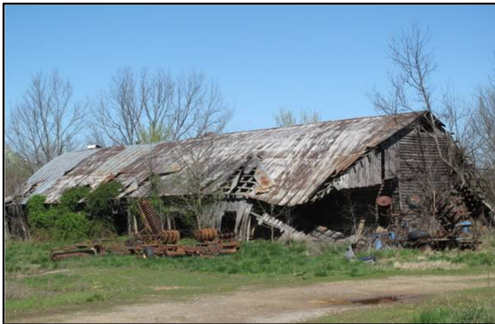
Figure 3. 67 South side of the corncrib at CN-32.
