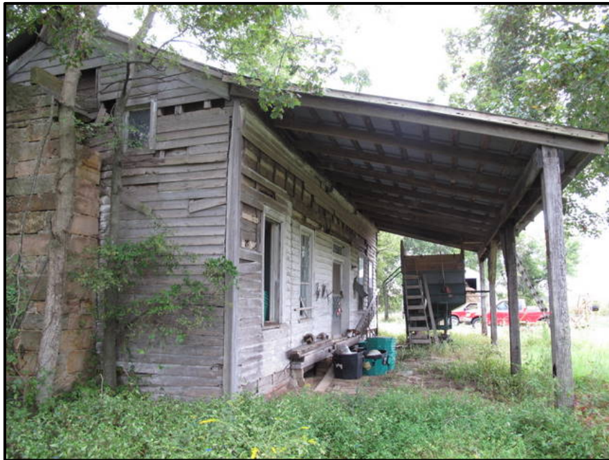
Figure 6. 11 The north gable end and façade of the Duley House, LV-81.
