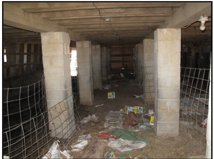
Figure 3. 30 Interior of the concrete block barn, CN-32, at the O.B. McDaniels Farm.
