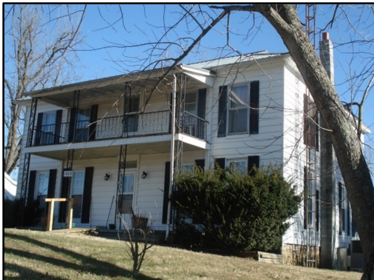
Figure 5. 20 Former Carrsville City Hospital (LV-114). Photo by Kathleen Guess.
