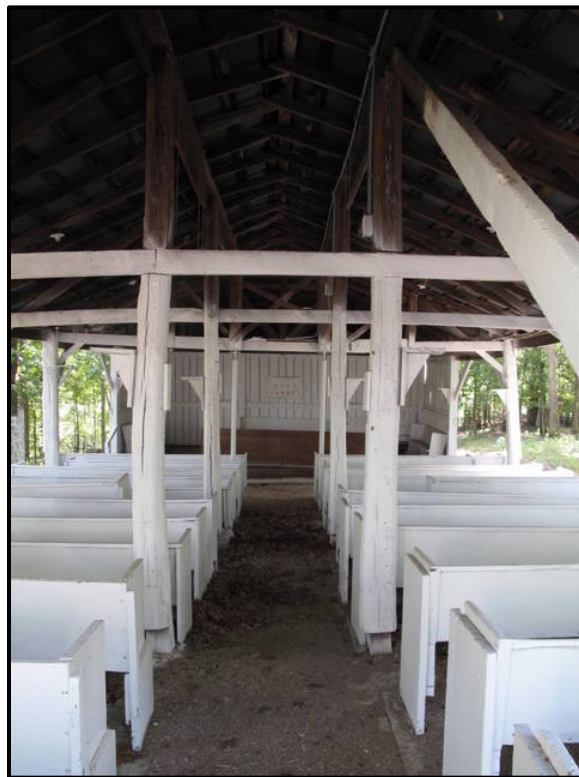
Figure 5. 37 Interior of shed at CN-68.
