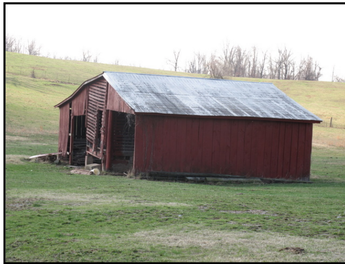
Figure 3. 70 Corncrib with side shed additions at LV-77.
